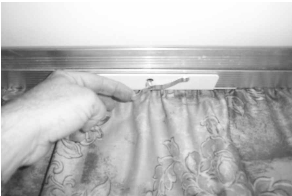
Release screen door from ceiling above door by pushing down on release pin and pulling door away from wall.
