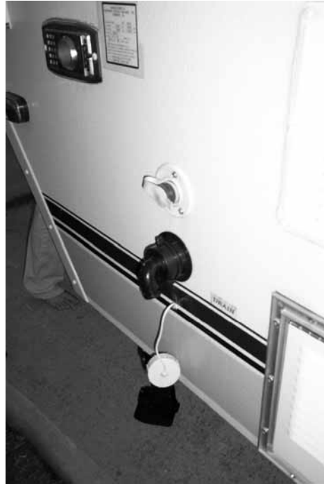
Sink Drains here, remove cap before using sink.
